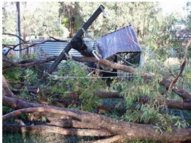
Images showing damage to the water pump station shed. The shed was hit with a tree and a power pole.
